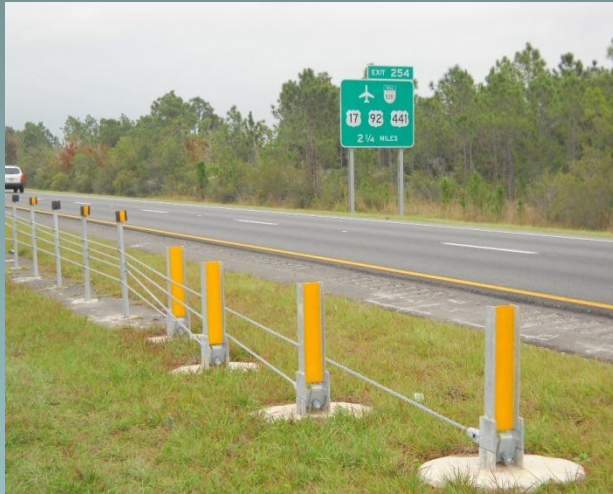
NUCOR Cable Barrier
