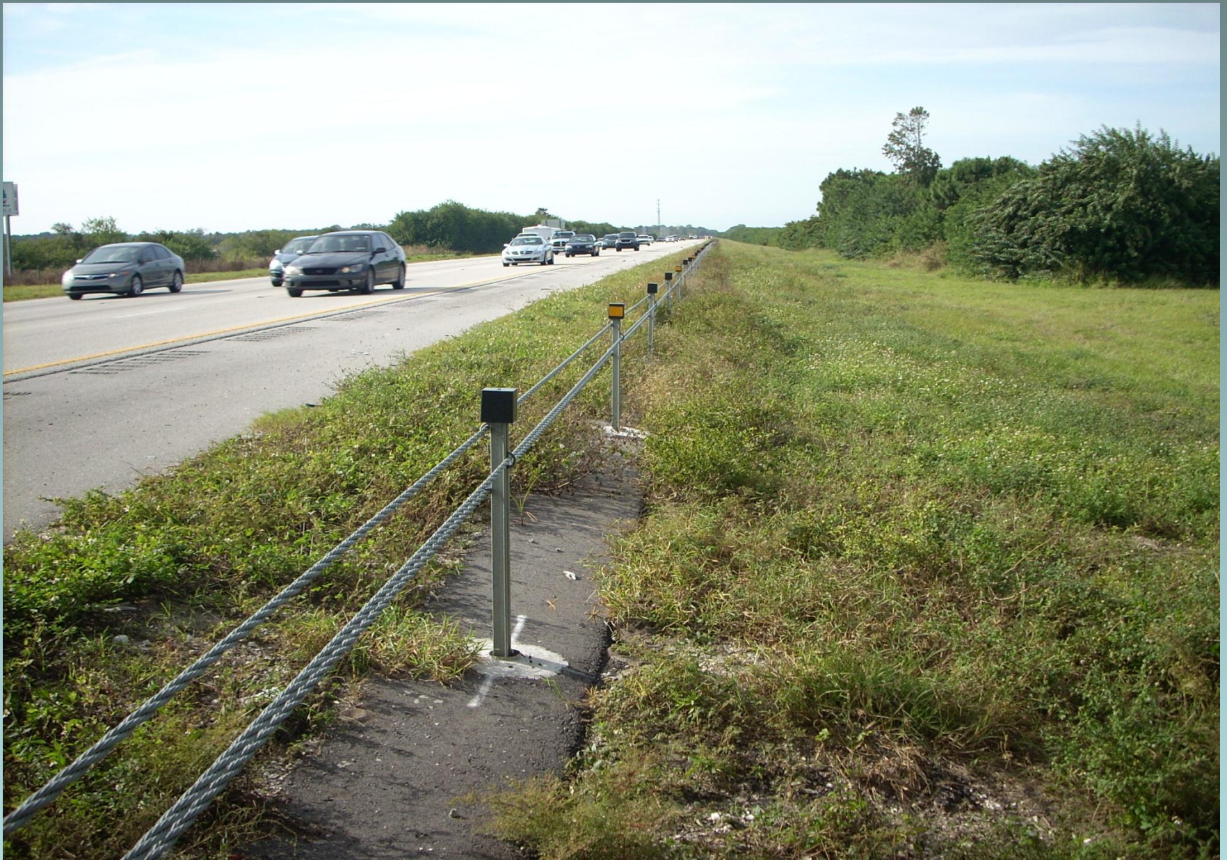
NUCOR High Tension Cable Barrier – I-75 & I-275, FDOT District 1
